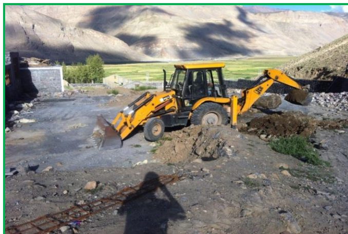
LEVELLING OF THE COMPOUND
