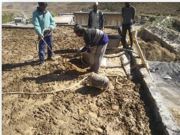
Applying a layer of mud on top of polyethylene sheeting
