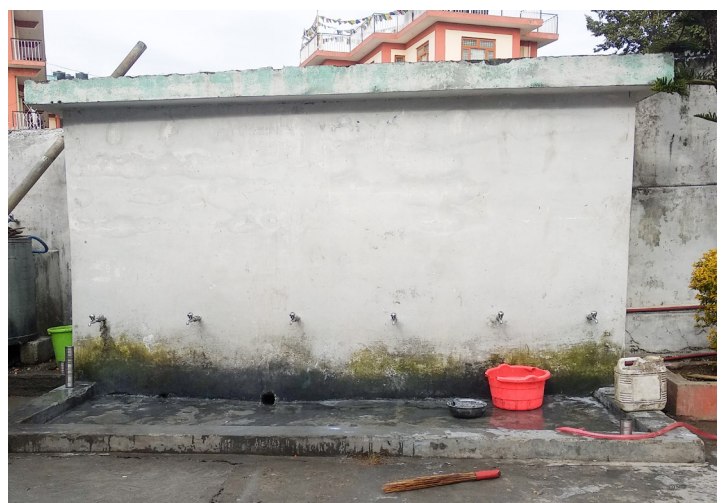
From GATE and Dr. Klauss we received a new water tank and washing station, which are presently used many, many times a day.
