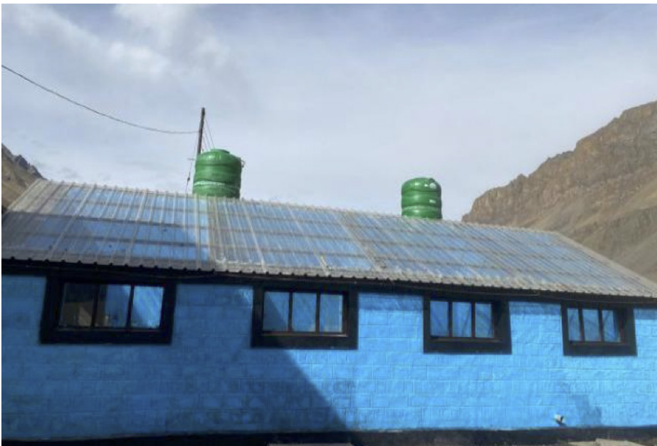
Translucent panelling on the roof at Rewa Primary School keeps the inside warm when the outside is freezing
