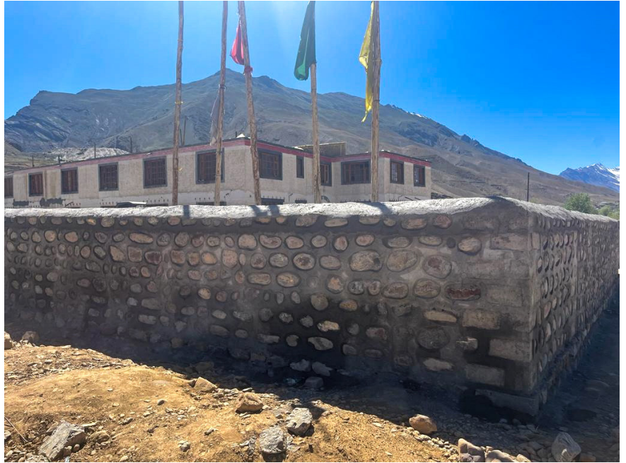
The new wall now in place at Rewa Primary School
