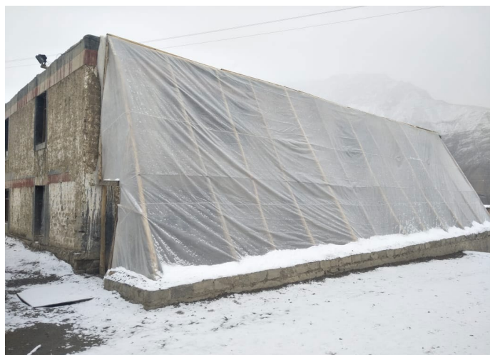
Passive solar heating with plastic sheets is inexpensive and very effective
